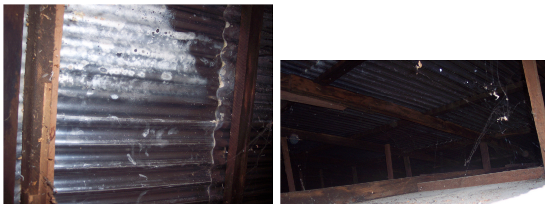
Figure 4 Wooden roof structure at MIA clinic
