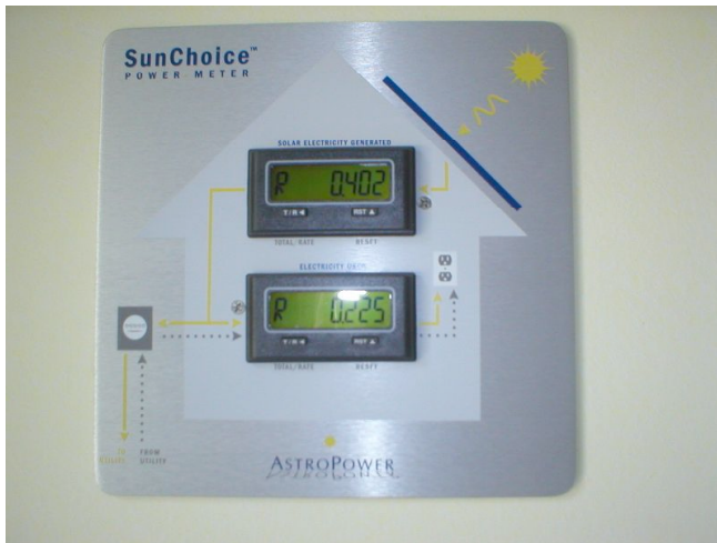
Fig. 5: Direct real time feedback of PV production and electricity consumption in Oberlin, OH. PV production is shown on the top, electricity consumption is portrayed on the bottom.
